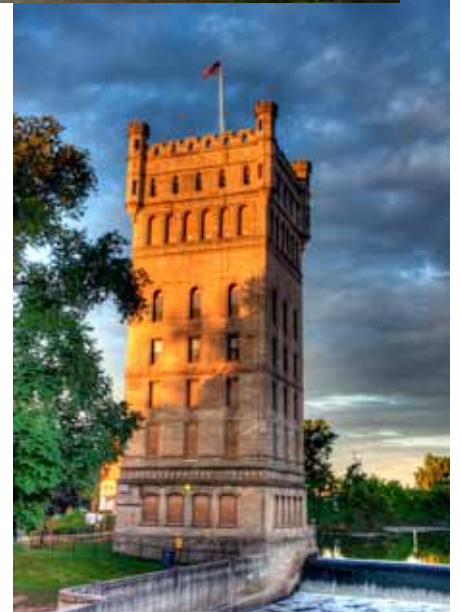
Hofmann Tower in Lyons, Photo by Dave Waycie
